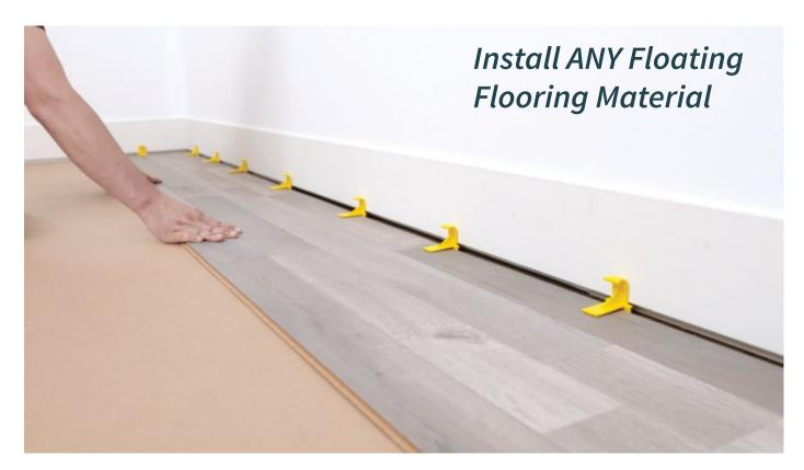
TFloor Spacers can be used to install any floating flooring material which requires an expansion gap of 1/4"- 3/8."
