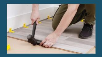
Even when tapping against it TFloor Spacers hold firm under pressure.
